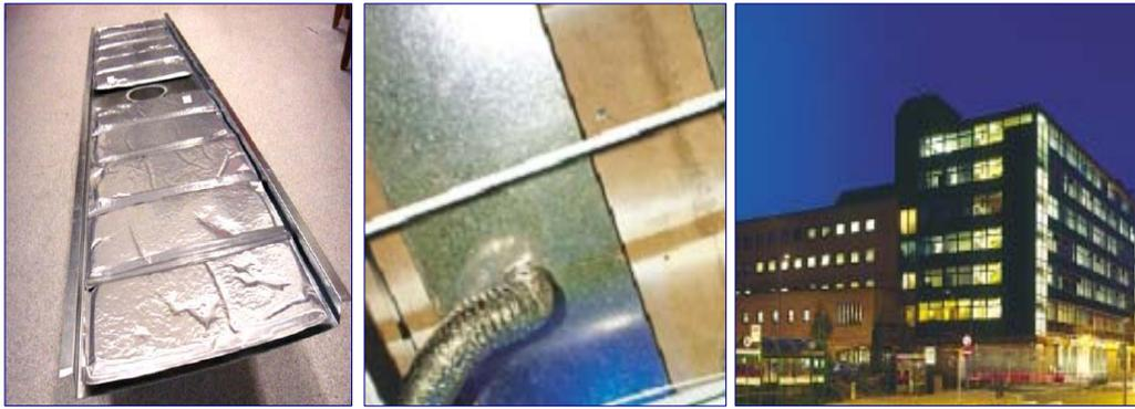
Figure 3-48 Picture of the "Stevenage Borough Council" building - construction details of the PCM based ceiling
