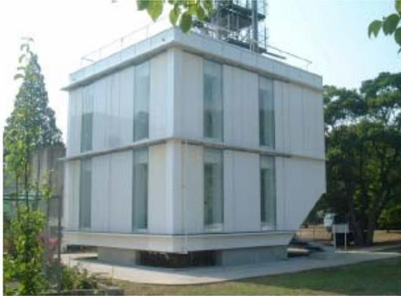
**Name of building:** Experimental Building with a Photo-Catalyst material coated facade
