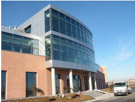
Building façade, East side
