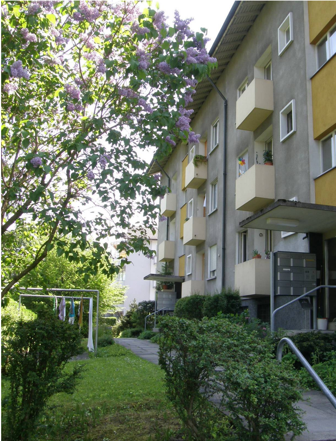
Northeast façade of case study building, Lucerne (see chapter 6.5), photo by R. Fischer, HSLU-CCTP
