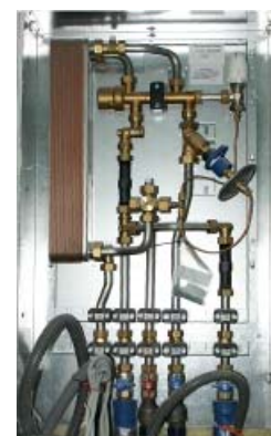
Figure 33: Transfer station installed inside a building
