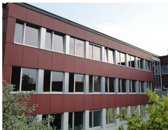
Figure 9: South-east oriented class-room windows – shaded with exterior blinds
