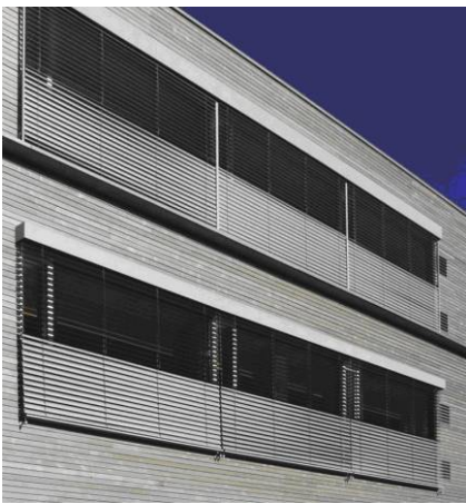
Figure 27: External venetian blinds, upper part adjustable for optimized daylight transport.
