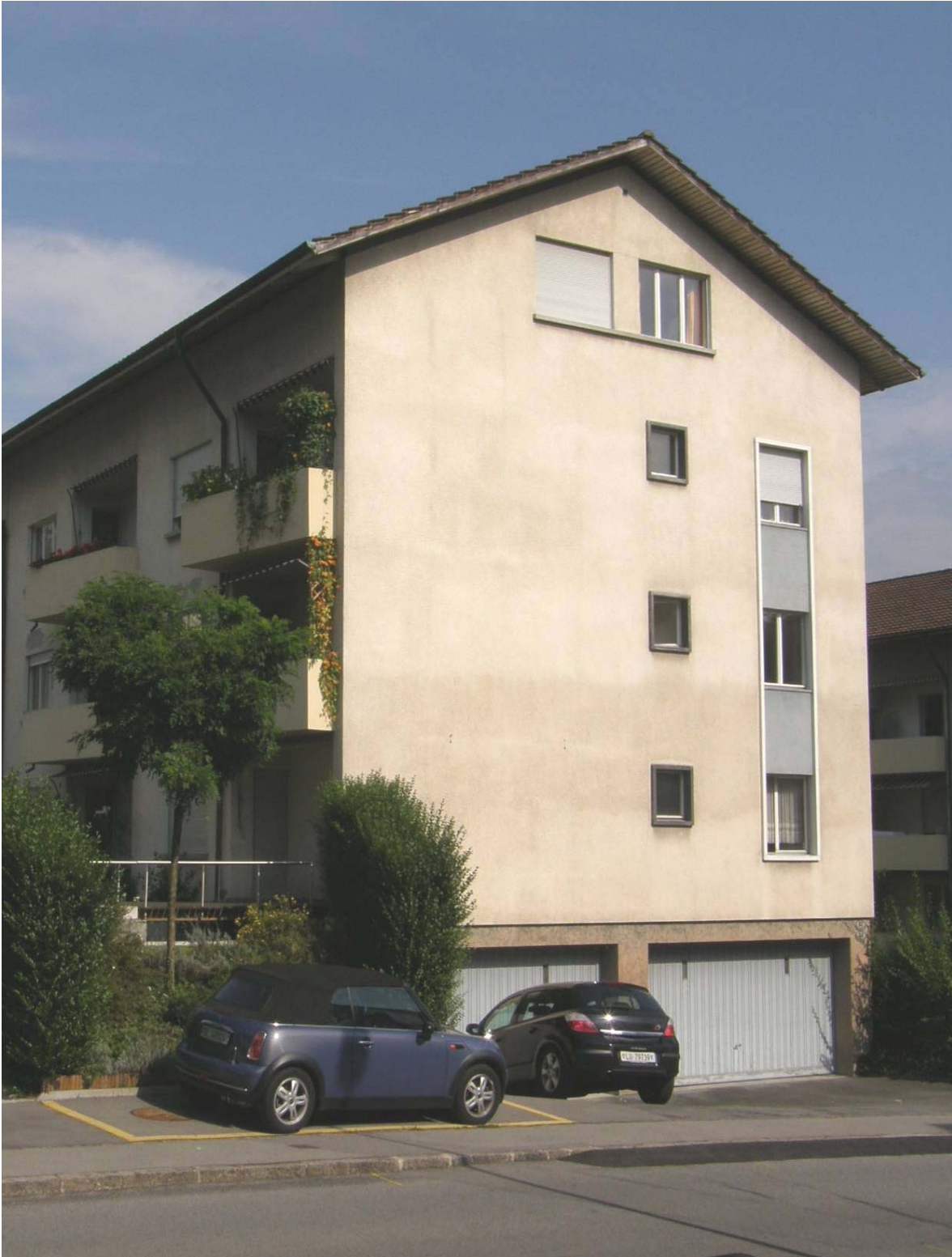
Northwest façade of case study building, Lucerne (see chapter 6.5), photo by R. Fischer, HSLU-CCTP
