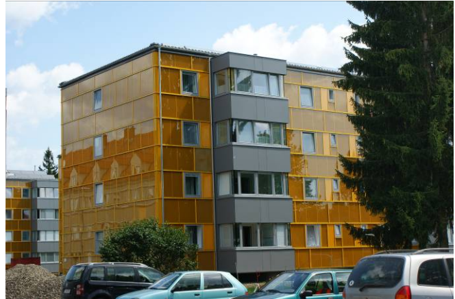
Figure 11: Integrated balconies after renovation within residential area Dieselweg, Graz
