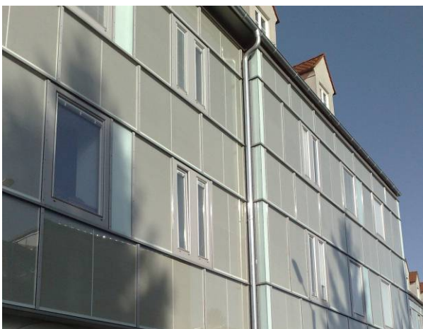
Figure 25: Windows exterior flush-mounted
