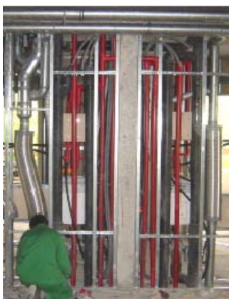
Figure 32: Installation module inside the building (Source: Ziv.Ing. Büro Boder)
