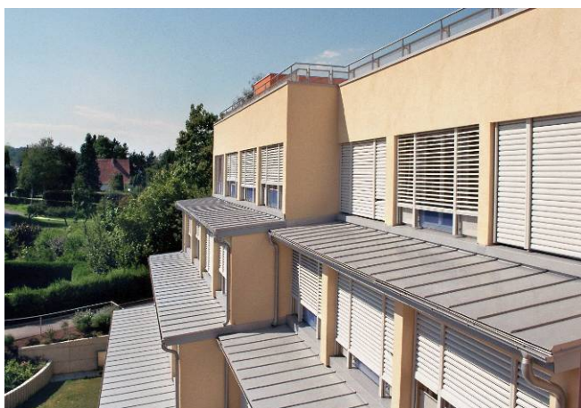
Figure 8: South-west oriented windows – shaded with exterior blinds (Source: Ziv. Ing. Büro Boder)
