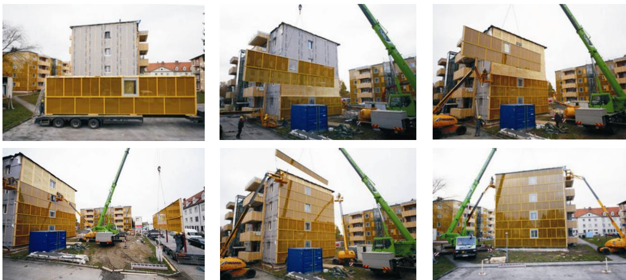
Figure 2: Assembling procedure of prefabricated façade modules within the renovation “Dieselweg”, Graz-Liebenau (Source: gap-solution)
