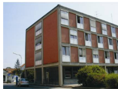
Figure 7: Building stock – skeleton construction (Source: LIG Steiermark)
