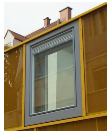
Figure 29: Blinds mounted "intermediate" (in-between the glass-panes) – to be used for plane façades.
