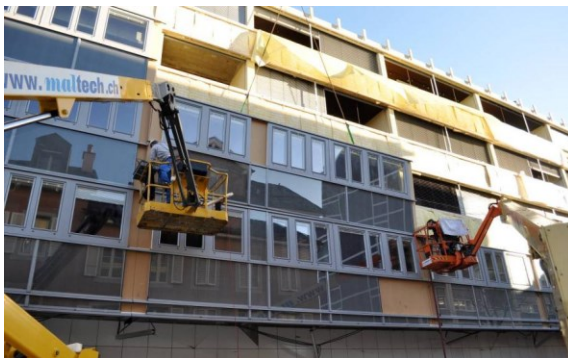
New prefabricated modules during the renovation
