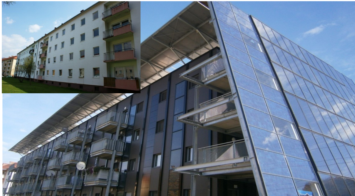
View of existing (small picture) and the renovated building (large picture) (west elevation)
