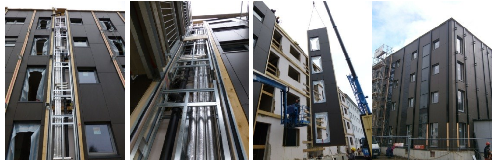
Different steps of the building renovation process: installation of the building services, assembling of the prefabricated façade modules, almost finished building envelope (f.l.t.r.)
