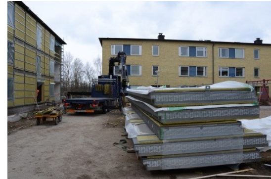
Prefabricated facade elements for the next phase of renovation.
