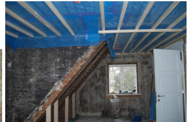
Below: The new vapour barrier on the loft
