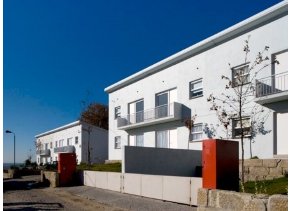
Front facade of the renovated buildings
