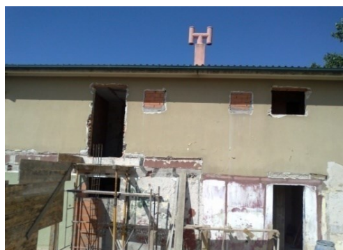
Building during the renovation process
