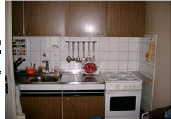
Kitchen before renovation
