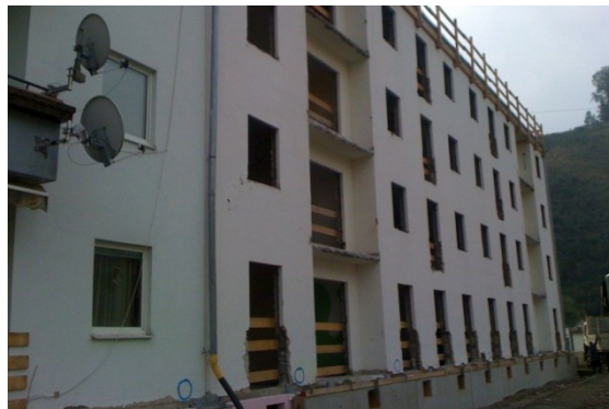
Façade during the renovation
