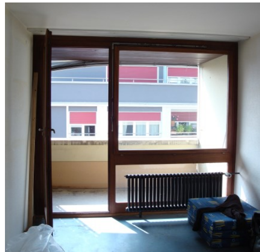
Living room before renovation
