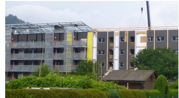
Left building part already renovated – right building part in the middle of the renovation
