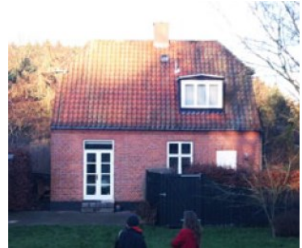
Above: Seen from the garden before renovation
