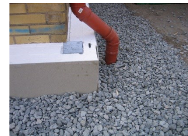
Added insulation to the foundation
