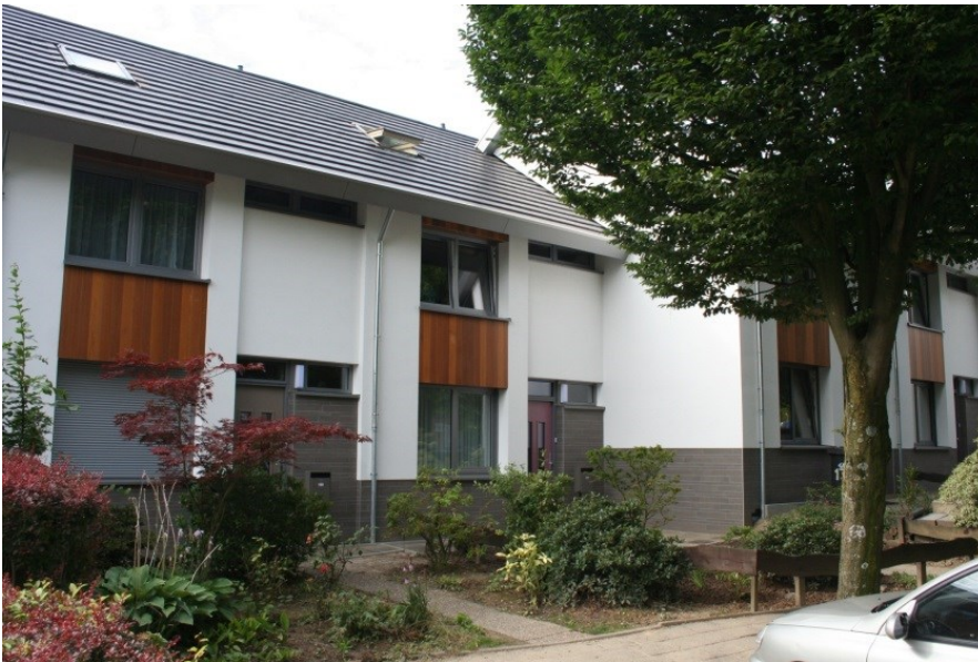
Figure: The houses after completion
