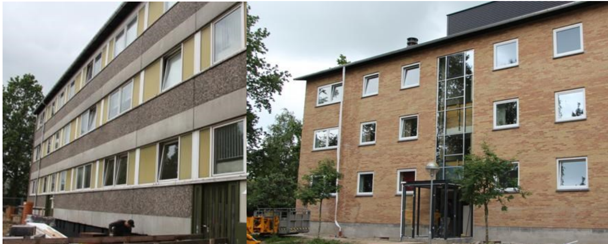
2 of the 3 blocks at Traneparken. The one on the left not yet renovated – the other after renovation.
