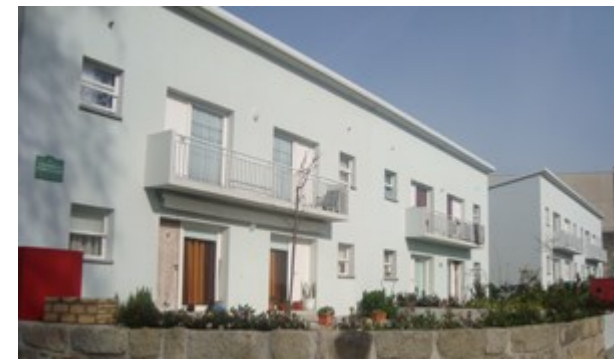
Building after the renovation process
