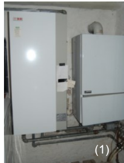
From left to right: 1. The old gas boiler and hot water tank. 2. Installation of the new B-labeled balcony door 3. Existing insulation in the loft
