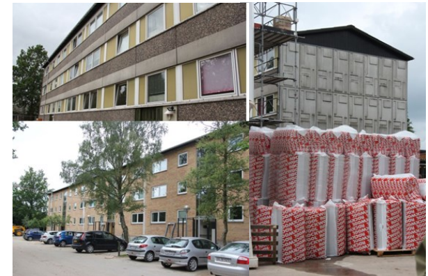
Facades – before and after:
