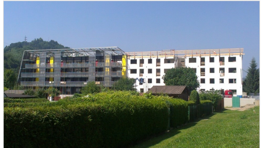
Left building part: finished renovation; right building part: still in renovation
