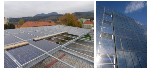
Mounting of the photovoltaic panels on the roof (left picture), pv and solar thermal panels on the south façade (right picture)
