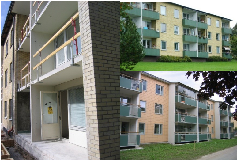
Long side façade with balconies before (left and above) and after (below) renovation.
