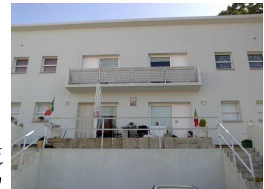
Above and right: Buildings after renovation
