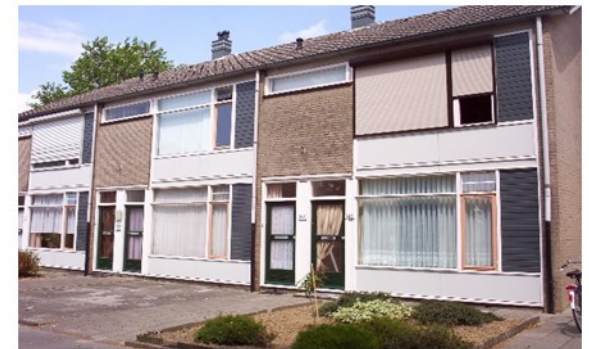
The houses before renovation
