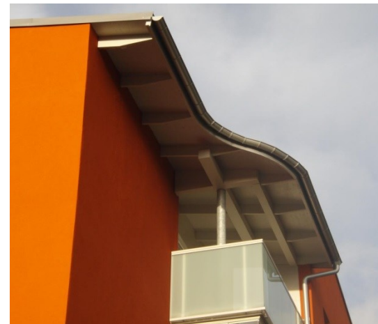
Extended eaves and balcony after renovation
