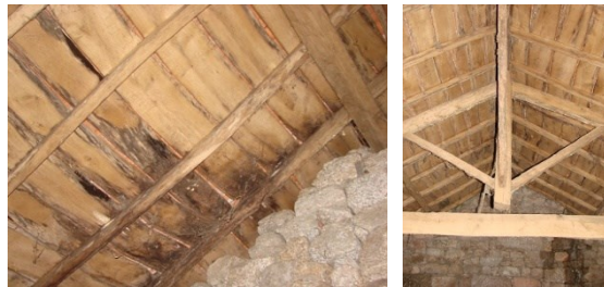
Roof condition and characteristics
