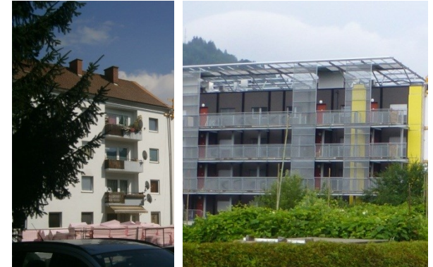
Facade – before and after the renovation
