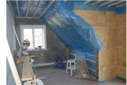
Insulation of mansard walls and lost space walls in attic incl. vapour barrier and internal insulation of the pediment
