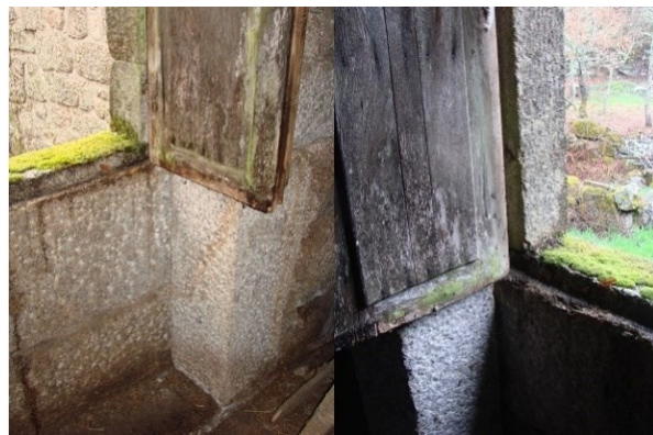
Existing window sills
