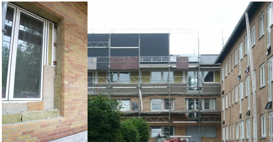
Figure: 190 mm insulation plus exterior solid standard bricks. Energy windows – aluminium – wood, 3-layer energy glass. In the panel walls: 285 mm insulation plus exterior solid standard bricks.
