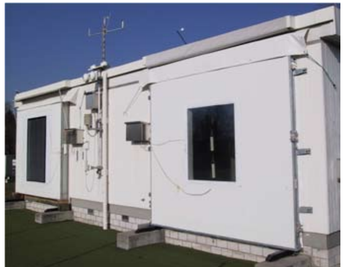
EMPA Test Cells, Exterior View.
